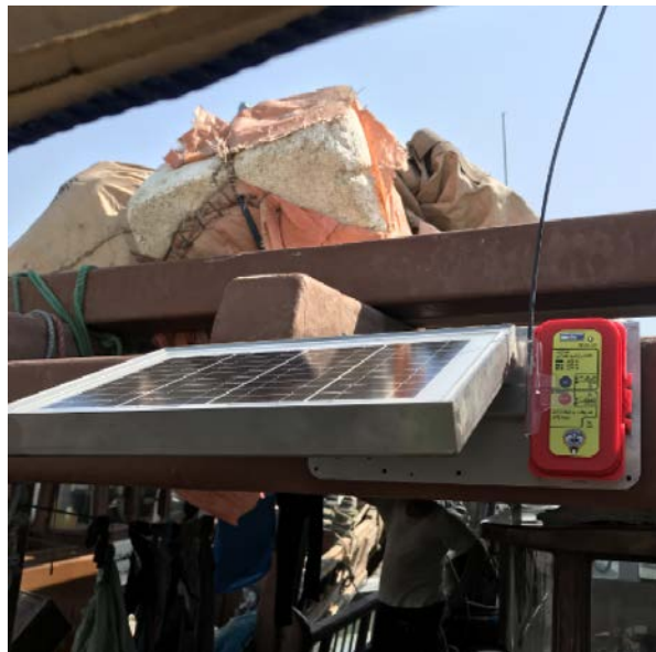
Figure 11: First position where unit was mounted
